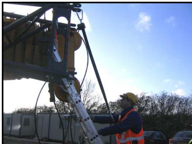
**Figure 3 - Fall Arrest System**
